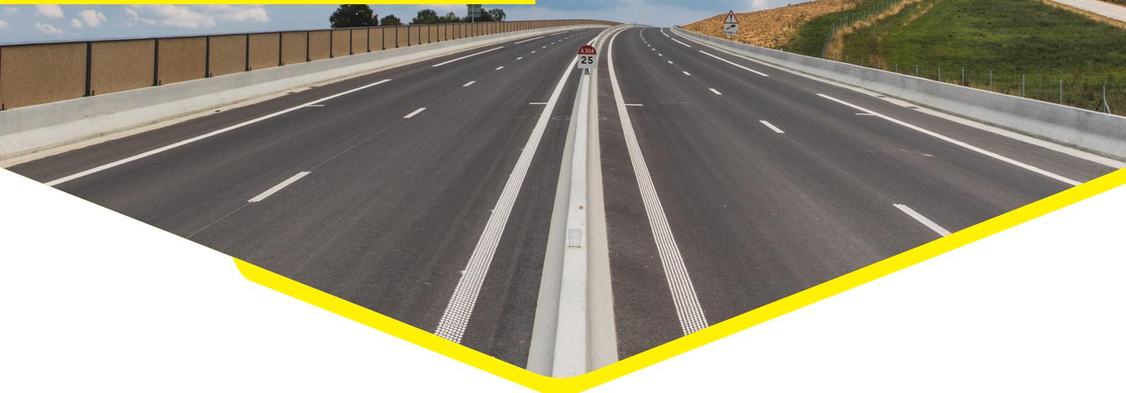
Coldraine is an open graded asphalt mix for roads bearing heavy traffic traveling at speed.
